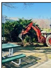
Overgrown Bush Removal Before
